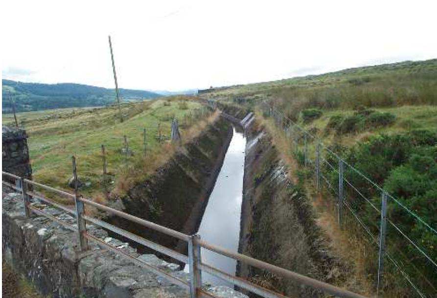
Figure 1.97: Ardudwy leat, between Cwrt weir and Crawwellt weir
