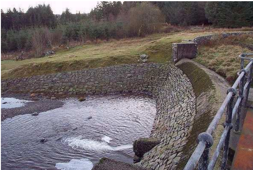
Figure 1.96: Downstream discharge into the Afon Cwrt
